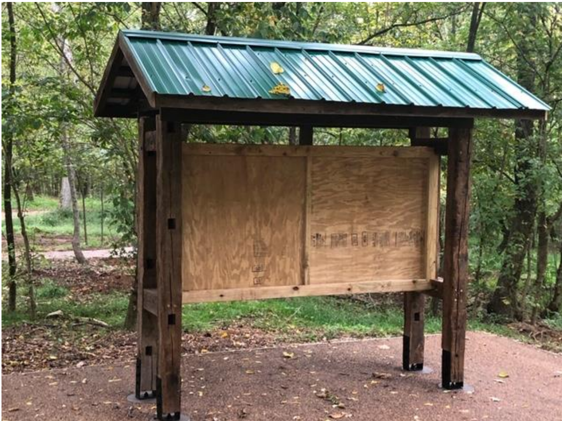
Kiosk built by Tony Headrick. Note PerkEPave material below kiosk.
